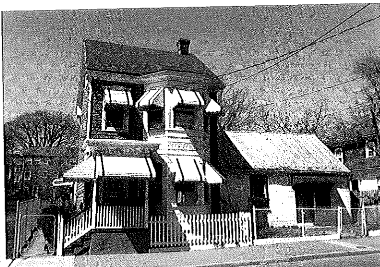
Figure 7 415 & 417 North Jonathan Street
